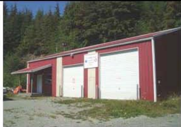
6. Emergency Services Building
