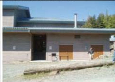
10. Boiler Room Lower Building
