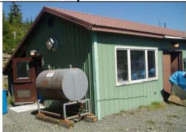
17. Water Treatment South Heater
