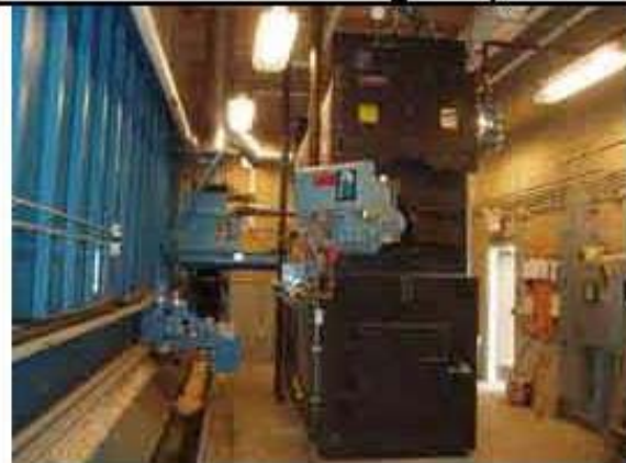
3. 4.9 MMBtuh Boiler Building Victor, MT
