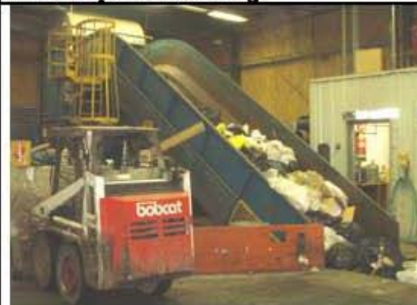
24. Waste Baler and Office
