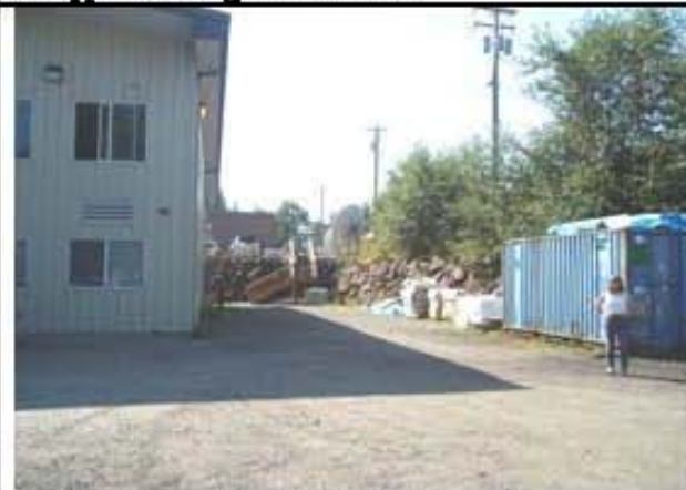
6. Road Access Possible Boiler Location
