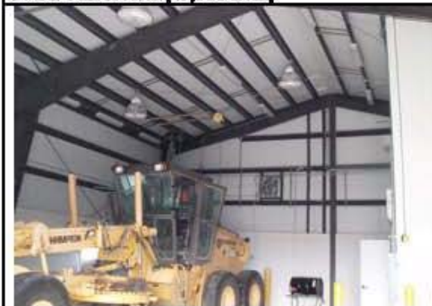
11. Heated Equipment Room
