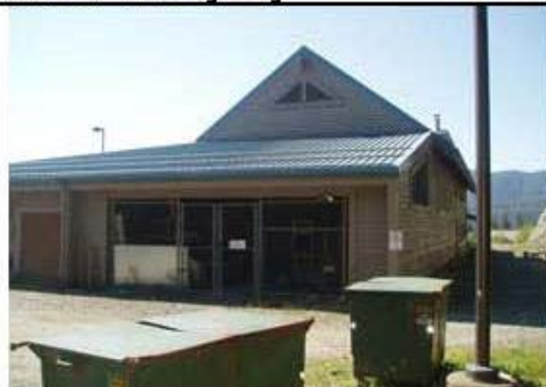
6. Back Wall to Upper Boiler Room
