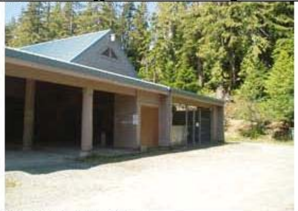
4. TB School Utility Entry
