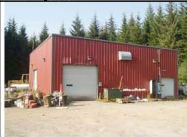
22. Municipal Waste Building
