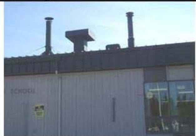
6. Existing Stacks and Vents
