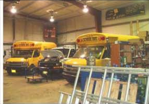
10. Air Heated Garage
