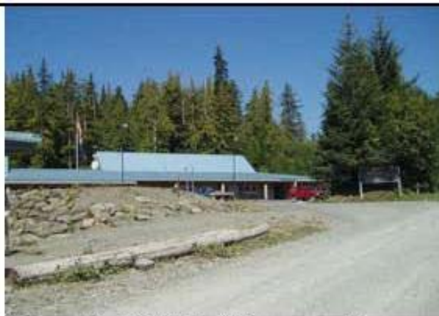
1. Thomas Bay High School Entry approach
