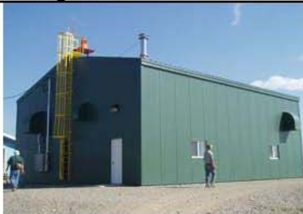
5. Unit Heater Stack, Rear Side
