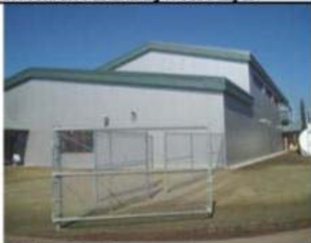
19. Side of New Elementary
