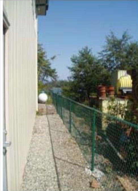
8. West Side Fence Line
