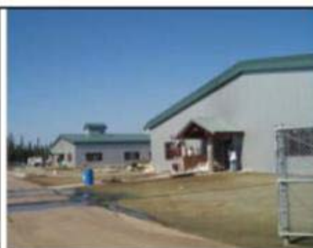
18. Front Entry New Elementary
