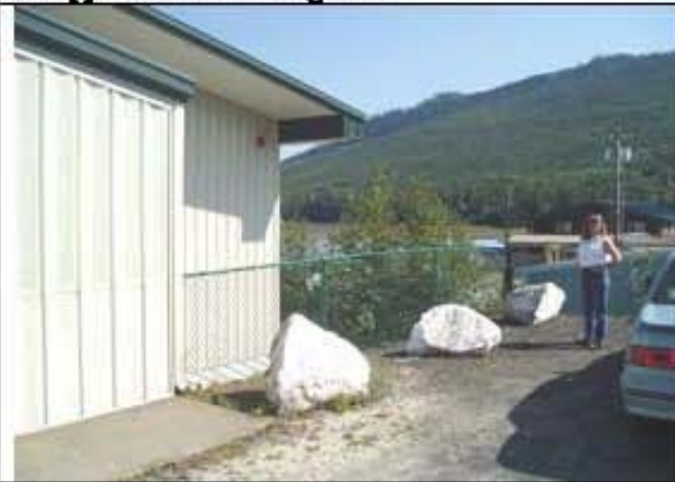
4. Upper Parking Above Boiler
