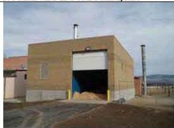
3. 4.9 MMBtuh Boiler Building Victor, MT
