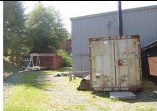
12. Access to Garage Air heater
