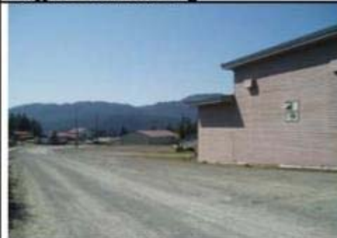
11. Road Past Lower Building
